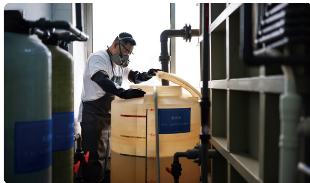
A worker is checking the conditions of the wastewater treatment device.
